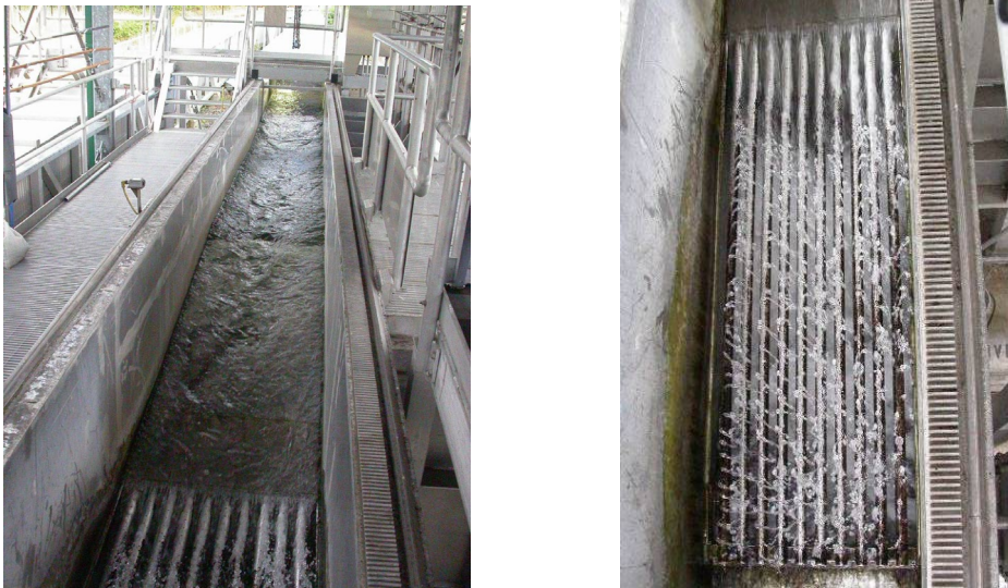
Figure 1. Primary Dewatering Structure (PDS) and the separator bars at the Juvenile Monitoring Facility.
